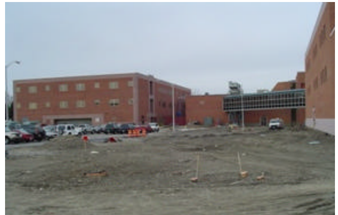
Surface Warfare Officers School Applied Instruction Building
